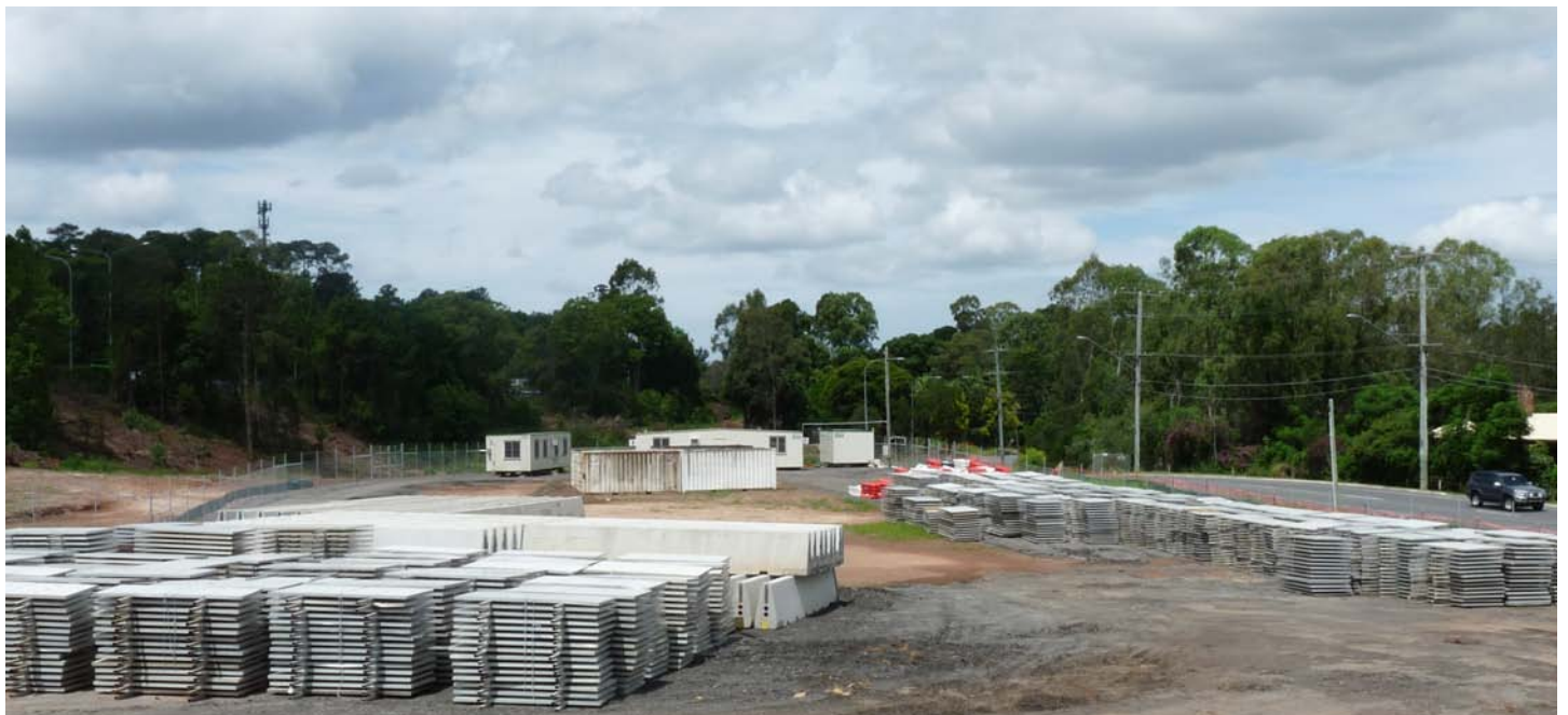
ABOVE: During the past month, tonnes of concrete traffic control barrier materials have been delivered to the temporary construction compound on Nujooloo Road at Slacks Creek. The concrete barriers will soon be assembled along the Pacific Motorway from Springwood (south) to Daisy Hill.
